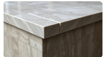
K.2 — SITE PHOTOGRAPH
