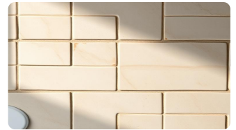
K.5 — SITE PHOTOGRAPH
