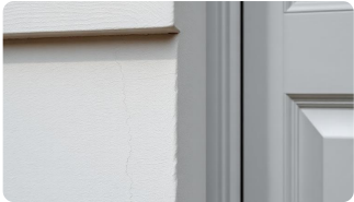
BE.1 – SITE PHOTOGRAPH
