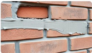
BE.3 – SITE PHOTOGRAPH
