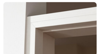
BS.4 — SITE PHOTOGRAPH
