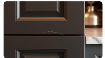
K.7 — SITE PHOTOGRAPH
