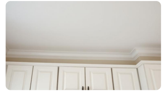
K.6 — SITE PHOTOGRAPH
