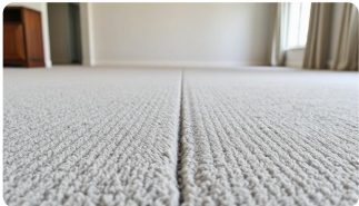
UR.3 – SITE PHOTOGRAPH
