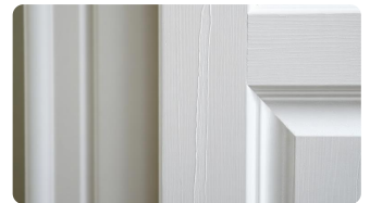
BS.6 — SITE PHOTOGRAPH
