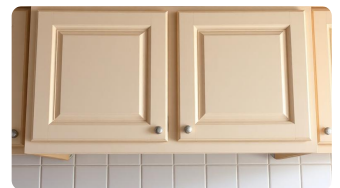
K.8 — SITE PHOTOGRAPH
