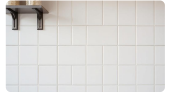
BS.1 — SITE PHOTOGRAPH
