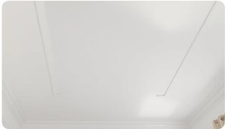
UR.1 – SITE PHOTOGRAPH
